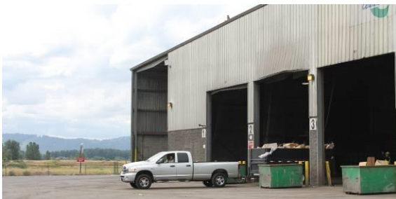
Haul waste to a transfer station.
